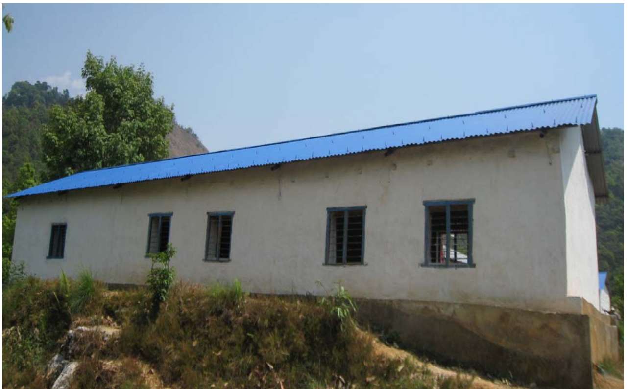
South side hut with 3 class rooms
