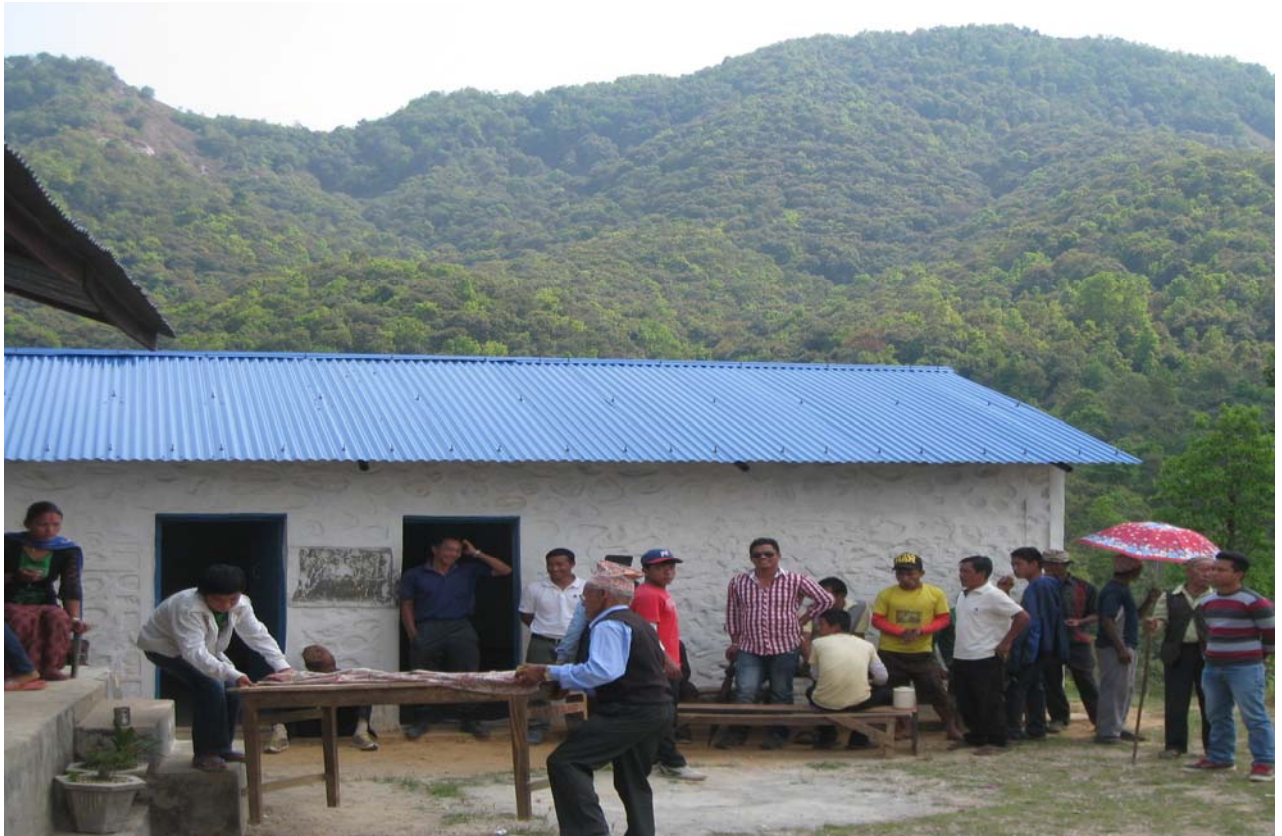
School with new CGI roof (North side school hut with 2 class rooms)
